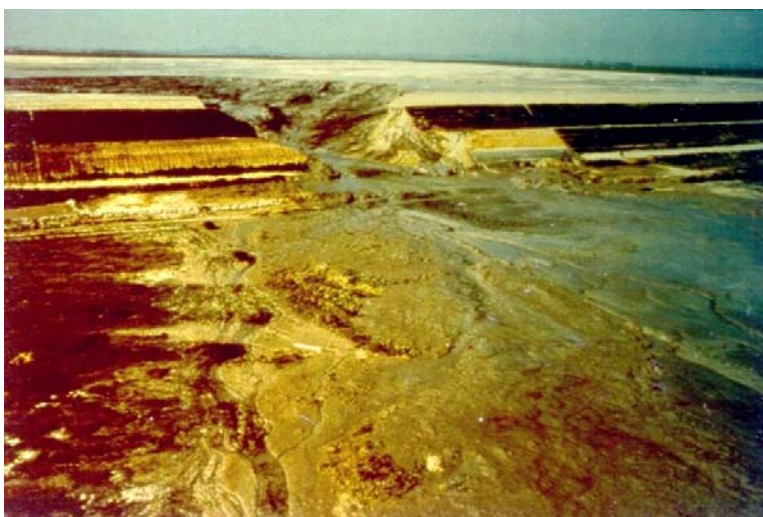
Figure 1: Failure of the Boliden lead-zinc tailings dam in 1998.
